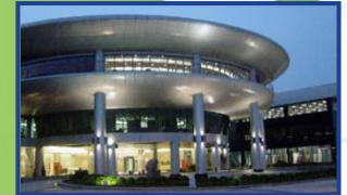
China Technology Center Shanghai, China
